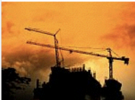
Crane On Tower In Construction
